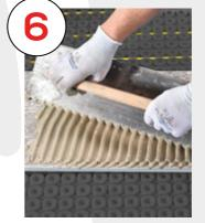
With the heating cable installed, you can apply a suitable adhesive (or self-levelling compound) and start laying the flooring. With the flat side of the notched trowel, fill the studs and cover the membrane with a suitable adhesive. Take care to cover the heating cable, the end cable connection and the floor sensor in the floor. Apply the adhesive with a notched trowel, appropriate to the tile size and lay the flooring.
