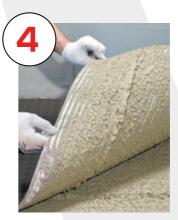
When laying the membrane, you must ensure there is adequate adhesive on the back and that it's fully covered. Peel back an area and if not covered in adhesive, apply as required.
