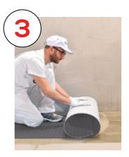
Apply the membrane, previously cut to the requirements of the room, pressing the membrane down immediately over the adhesive and apply pressure using a roller or trowel.
