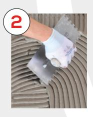
Using a 6mm notched trowel spread a substrate compatible flexible tile adhesive over the substrate.
