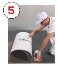
Lay the next sheet of membrane taking care to align it with the previous one, without overlapping. Align the square studs to enable the cable to be installed. Repeat previous steps until the room is covered in membrane as required.
